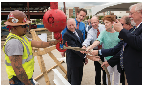
Hospital and community leaders help prepare the final beam to be placed atop a second professional office building, to be completed in spring 2018. The four-story building is the first to be built on the hospital's southwest campus.
